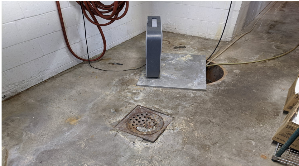
SUMP AND FLOOR DRAIN, SITE STRUCTURE BASEMENT.
