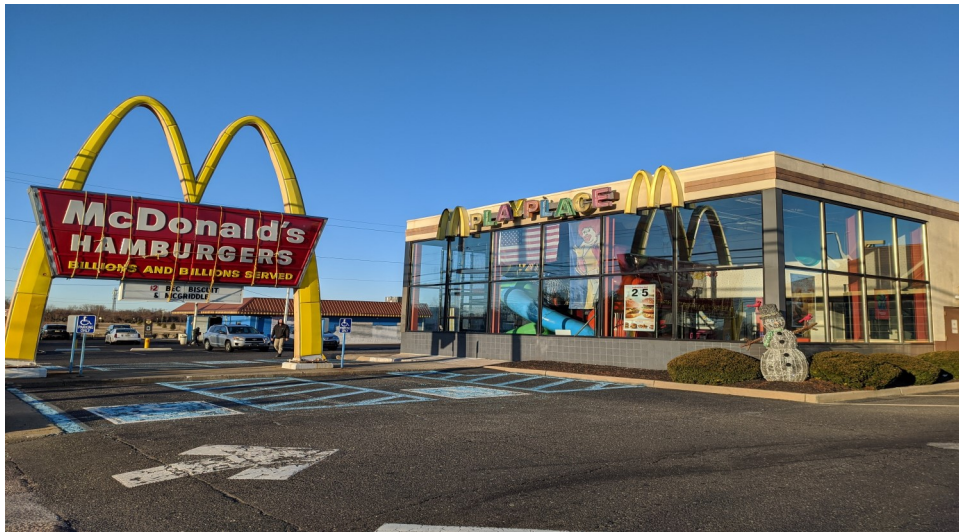
SITE STRUCTURE, VIEW TO THE WEST.
