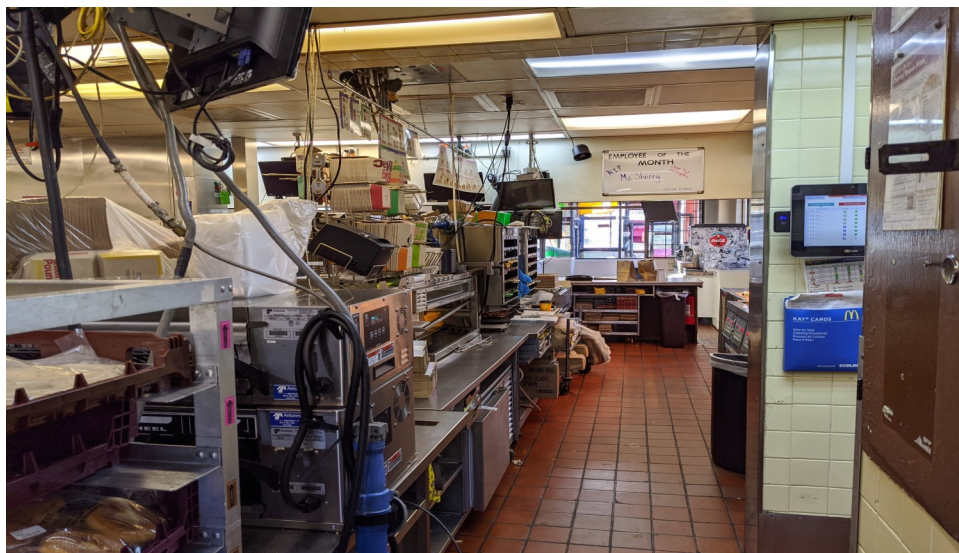
SITE STRUCTURE, KITCHEN INTERIOR.
