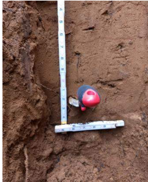
Photo 2: TP6 Lower Side Wall Looking Southeast
