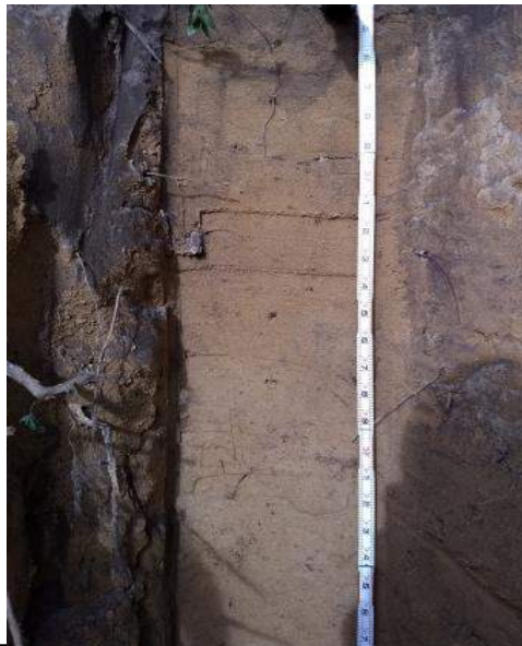
Photo 2: TP4 Northwestern Side Wall
